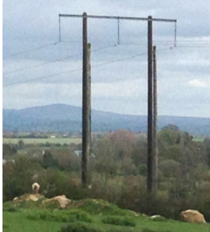
Figure 4.5: Example of existing 110 kV poleset being replaced with new and in this instance taller poleset (old poles still to be removed)
